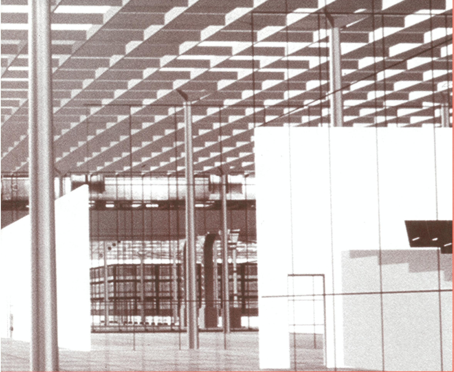
Columns in the Jahn/Sobek scheme are tapered steel tubes with supporting cross arms at slab locations and at the roof grid mesh. The center is designed "to highlight in an architectural setting the research interests of the schools of engineering, thermodynamics, materials research, performance of fabrication . . . within the design of the dynamic and technically advanced building envelope."
